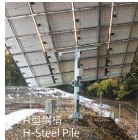
駆動基礎 Driven Piling
